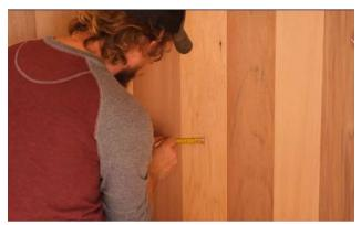
On the center of the back wall, measure 22" (56mm) from the floor up.
