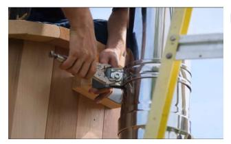
Reassemble the top chimney support bracket.
