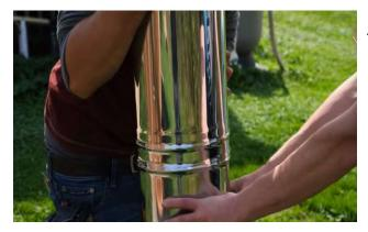
Assemble together the remaining chimney pieces.
