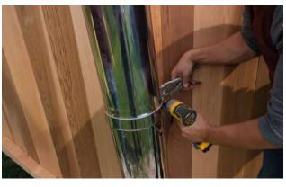
Attach a support strap around the connection and tighten up.
