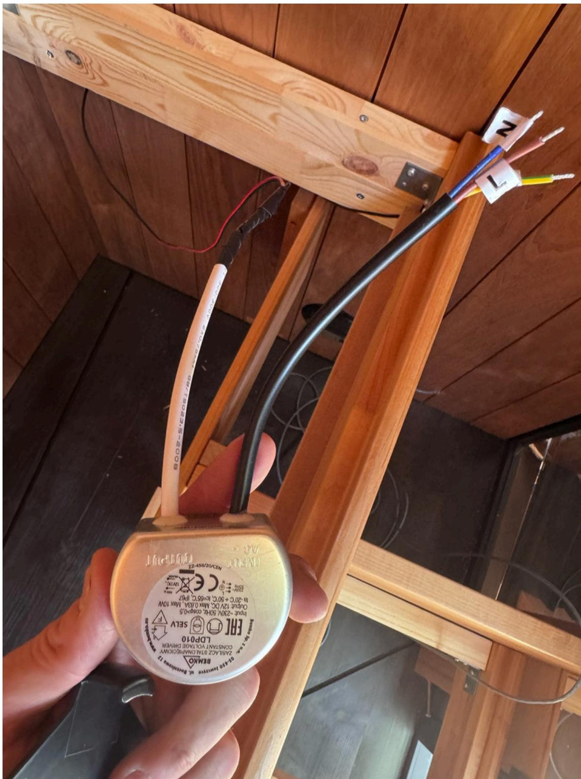
THE DRIVER CAN BE MOUNTED UNDER THE BENCH USING A CABLE TIE. IT'S IMPORTANT TO USE WATERPROOF CONNECTORS (BUTT SPLICE OR WIRE NUT).
