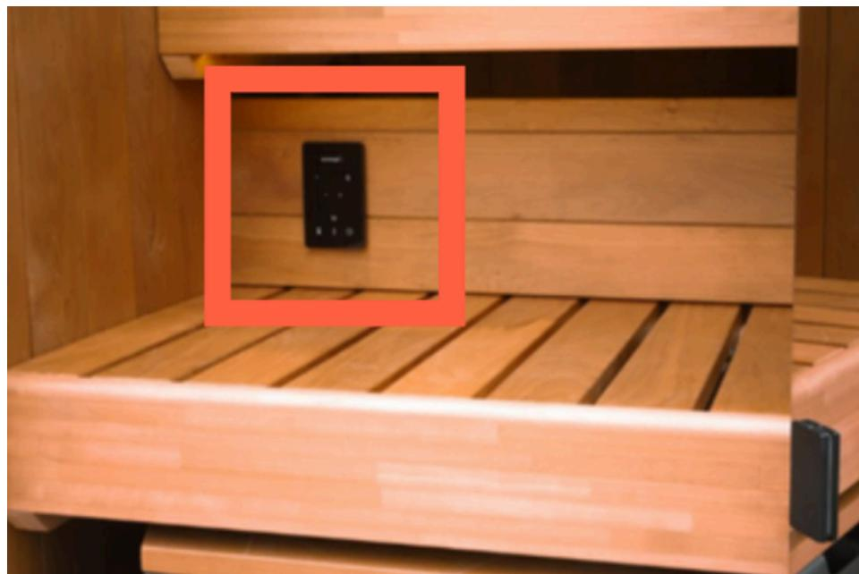
**THE TEMPERATURE SENSOR WILL BE INSTALLED ABOVE THE HEATER. THERE IS A PRE-DRILLED HOLE FOR THE 2 CONDUCTOR WIRE TO BE RUN WITH A PULL WIRE LOCATED AT THE BASE OF THE WALL:**
