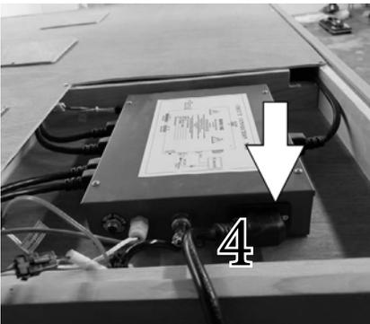
5. Replace the top panel screws and feed the power cable through the hole.
